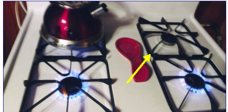
Igniter did not function and should be repaired at the top right burner. We recommend further evaluation and service.
