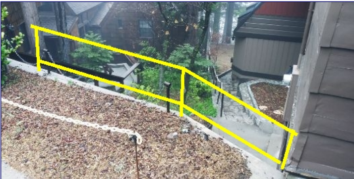
We recommend installing a handrail system where a drop in elevation of 30" or more is present at known paths of travel, as local building standards would require. We recommend further evaluation and service.
