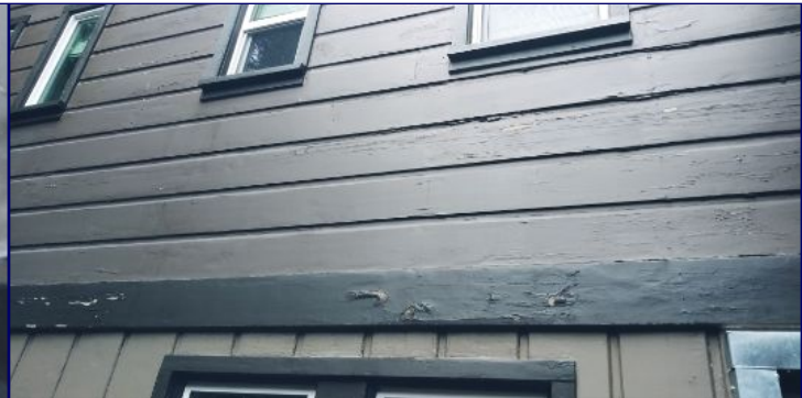
Peeling paint present and we recommend service. Homes constructed pre 1978 to 1982, lead based paint is likely to be present and testing should be done to determine for certain. If the presence of lead is confirmed the painting, paint prep, and/or paint removal should be completed by a licensed painting contractor who holds a certification in handling and servicing lead based paint.
