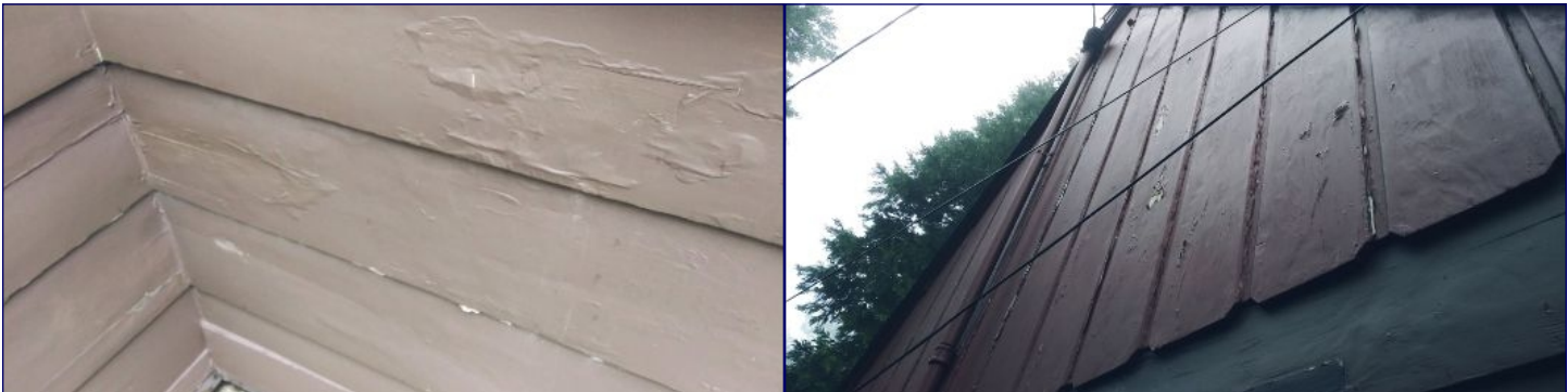
Peeling paint present and we recommend service. Homes constructed pre 1978 to 1982, lead based paint is likely to be present and testing should be done to determine for certain. If the presence of lead is confirmed the painting, paint prep, and/or paint removal should be completed by a licensed painting contractor who holds a certification in handling and servicing lead based paint. Peeling paint present and we recommend service. Homes constructed pre 1978 to 1982, lead based paint is likely to be present and testing should be done to determine for certain. If the presence of lead is confirmed the painting, paint prep, and/or paint removal should be completed by a licensed painting contractor who holds a certification in handling and servicing lead based paint.
