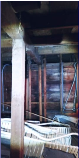
Leaning and off center structural support posts are present and should be serviced as soon as possible. Leaning posts indicate considerable movement due to structural failure and we recommend further evaluation and repair prior to occupancy. Furthermore beam transitions are not properly supported by a support post and we recommend service.
