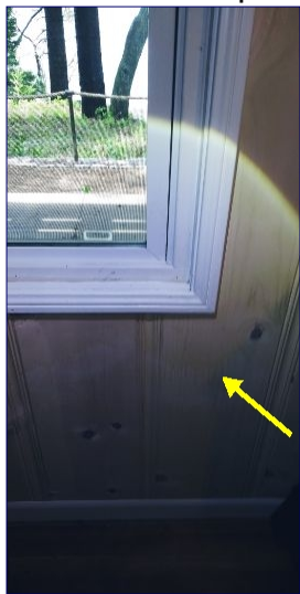
Visible moisture related damages present beneath the window sill within bedroom three. We recommend further evaluation and service.
