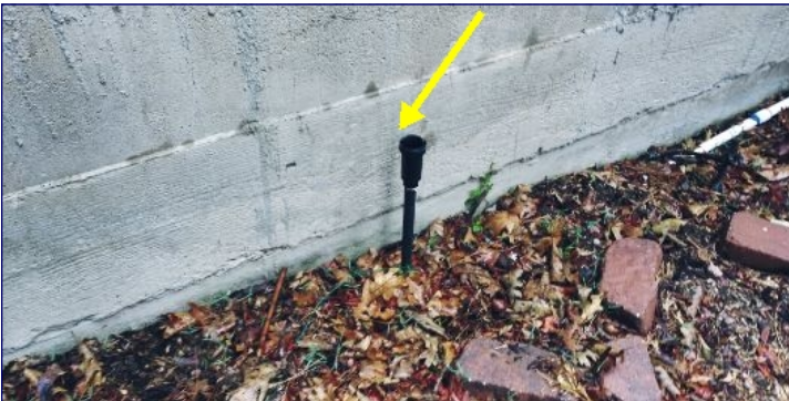
There are missing or broken sprinklers and we recommend service.
