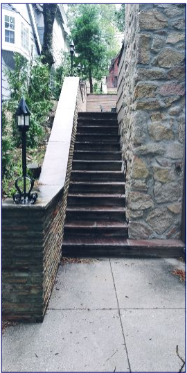
There should be a graspable handrail installed where there is three or more risers and we recommend service.
