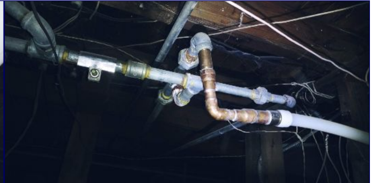
There are surface-mounted water pipes that are not insulated and are therefore not energy efficient and if location warrants, will be susceptible to freezing, and you may wish to verify the installation permit.
