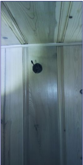
Missing trim, loose, and/or damaged trim at various locations
