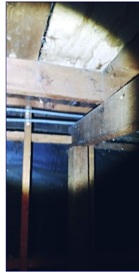
Load transfer missing at joist to cripple wall connection within the main foundation crawlspace at one or more locations. We recommend further evaluation and service by a licensed structural engineer.
