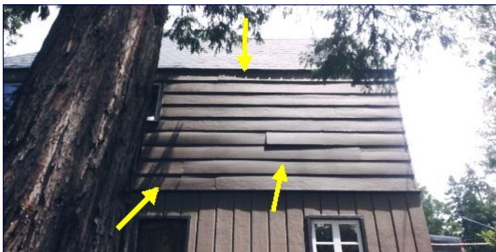
Loose siding present at multiple locations and we recommend service.
