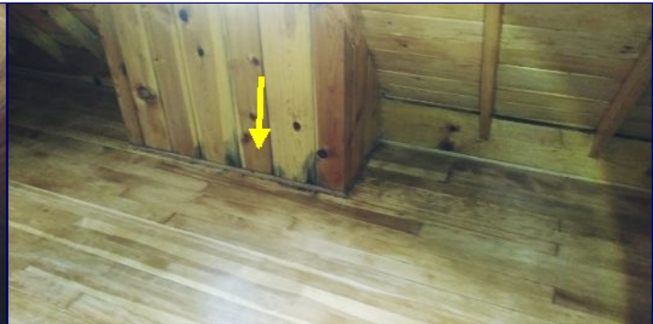
Moisture related damages are present at the base of the wall within the interior of the main structure, off the top floor bedroom areas. We recommend further evaluation and service by a licensed moisture intrusion specialist.
