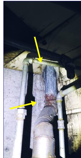
Moisture related damages are present at the vent pipe for the water heating unit which services the detached structure. We recommend further evaluation and service prior to any further attempts to use.
