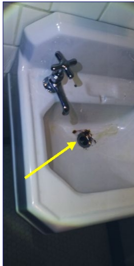
Damaged sink present within bathroom two. We recommend further evaluation and service with the intention of replacement.
