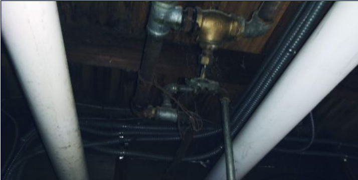
There are blisters on the body of the galvanized water pipes that should be evaluated
