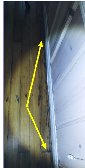
Visible moisture damages are present at the base of the wall and ceilings within the sublevel den. We recommend further evaluation and service by a licensed moisture intrusion specialist.
