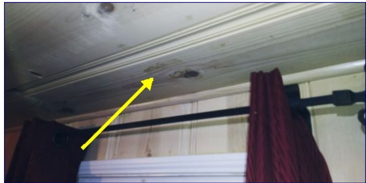
Visible moisture damages are present at the base of the wall and ceilings within the sublevel den. We recommend further evaluation and service by a licensed moisture intrusion specialist.
