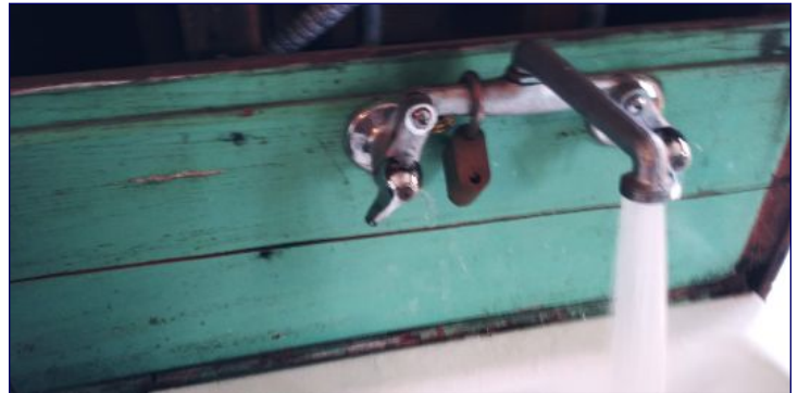
Visible leaking at the water mixing valve located at the laundry sink, within the detached structure. We recommend further evaluation and service by a licensed plumbing contractor.
