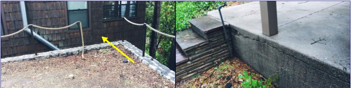
Sections of rope style railing are damaged and/or missing at one or more locations. We recommend further evaluation and service.
