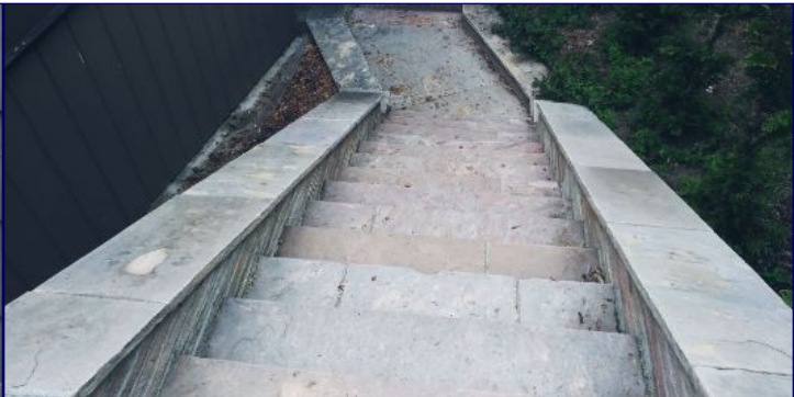
There should be a graspable handrail installed where there is three or more risers and we recommend service.
