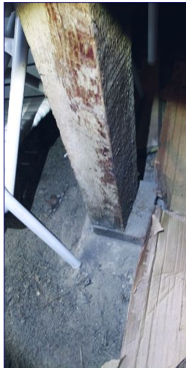
No structural/seismic hardware connections at post to beam connections
