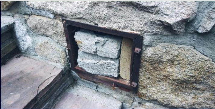
Missing ash box door and we recommend service prior to any attempt to employ system.
