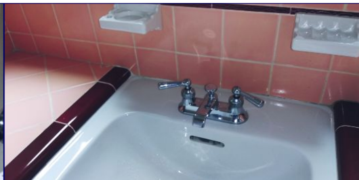
One or more faucets leak when in use. We recommend further evaluation and service by a licensed plumbing contractor.
