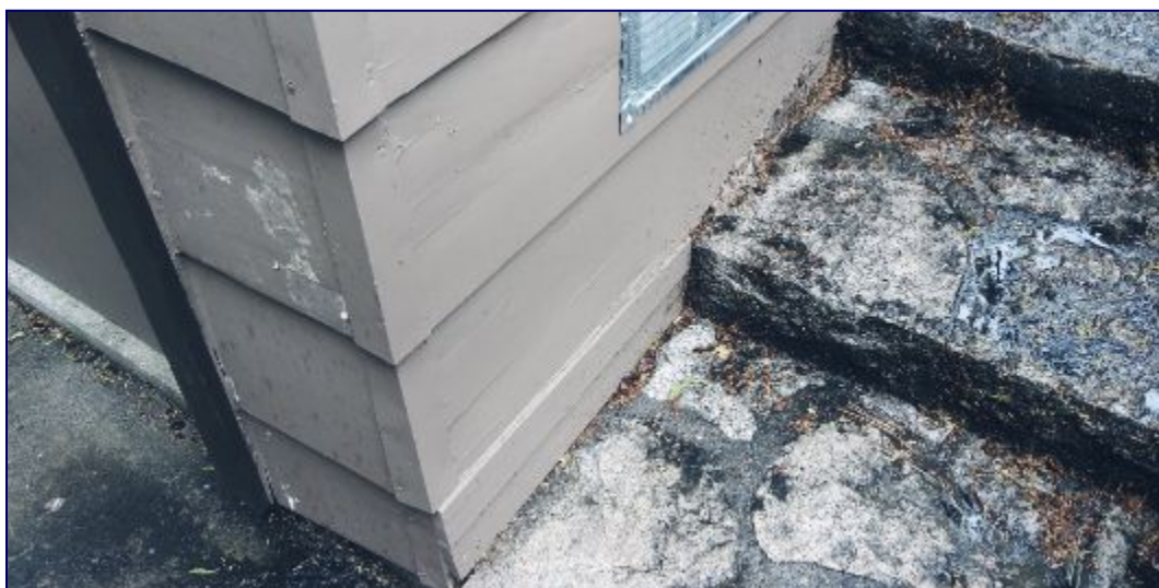
Wood siding is ran into the concrete and/or dirt, which will promote rot and termite infestation. Local standards require a 4" separation when dirt is present and 2" when concrete is present. We recommend further evaluation and service.
