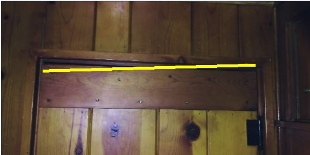
Multiple uneven door reveals present, indicating out of square openings.
