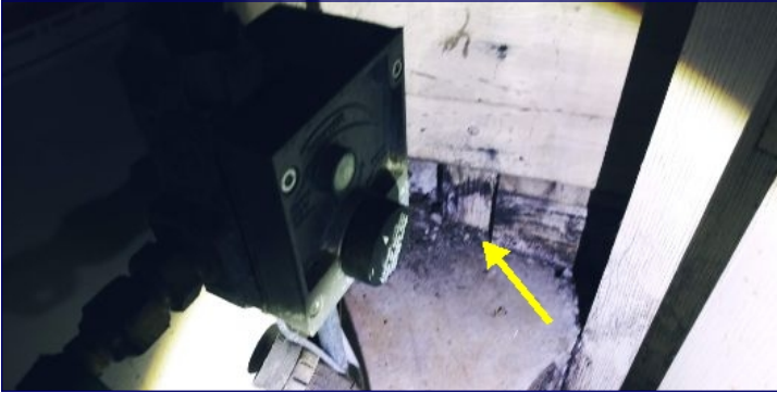
Deteriorated materials present at the water heater enclosure and/or access door and we recommend service.
