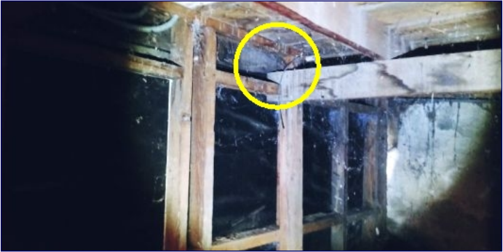
Load transfer missing at joist to cripple wall connection within the main foundation crawlspace at one or more locations. We recommend further evaluation and service by a licensed structural engineer.
