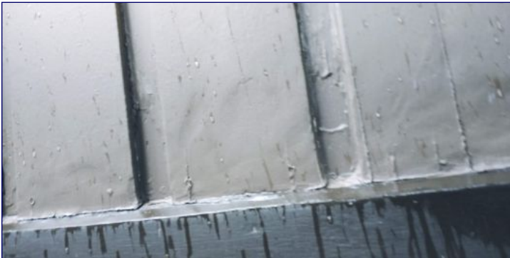
Sections of the fascia board or wood trim are weathered
