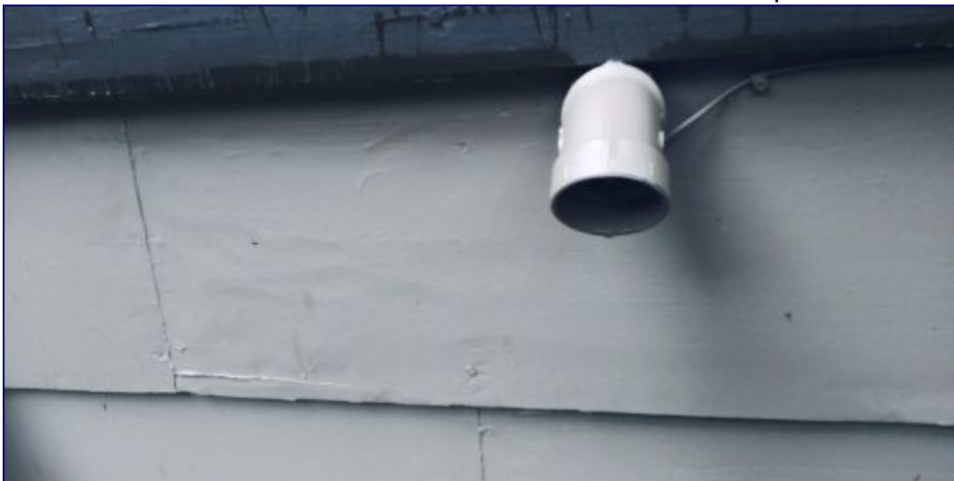
The termination method is improper and missing a screened port to prevent access to rodents at the water heater vent located beneath the main house off the left elevation. We recommend further evaluation and service.
