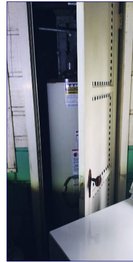
At the water heater located within the guest house, we have noted the combustion air available to the water heaters is inadequate, due to the undersized ventilation grates and the under sized bathroom those greats are attempting to draw combustion air from. We recommend the water heaters not be employed until properly serviced by a licensed plumbing contractor.
