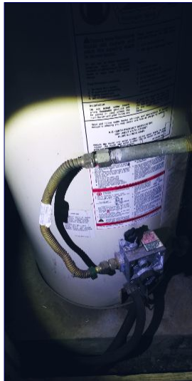
Sediment trap missing at the gas supply line and we recommend service.
