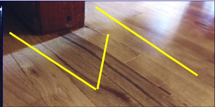
There are abnormal and significantly uneven areas in the flooring, ceilings, and interior door openings were found to be present at one or more locations within the foyer, dining room, and main hall locations. We highly recommend further evaluation and service by a licensed structural engineer prior to the close of escrow.
